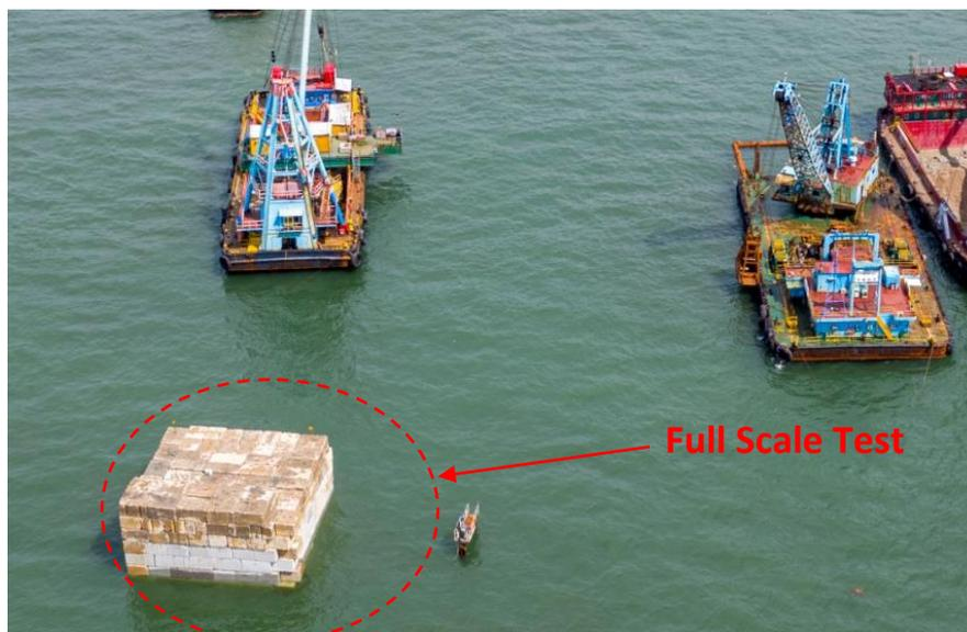
**Plate 1** - Site Photo of loading concrete blocks
